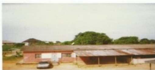
Figure 2(a) Outside view of Site C1
