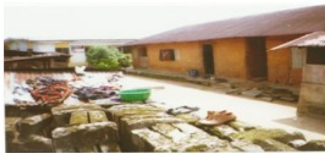
Figure 4(a) Outside view of Site M1
