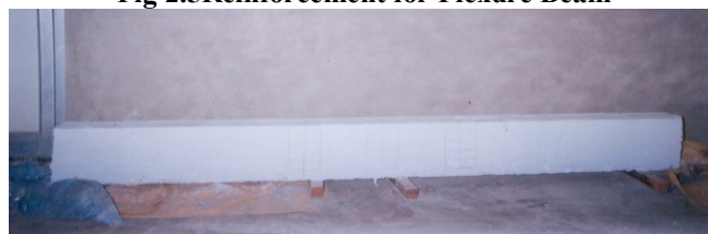
Fig 2.6 Beam after casting
