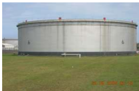
Figure 1: Reservoir at the Terminal
