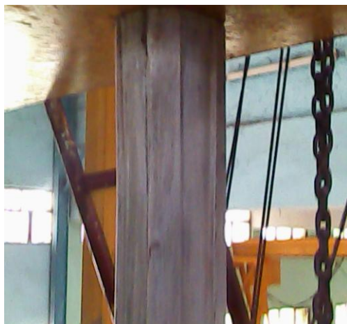
4(c) Failure of column L/D 25 at top with 3/#8
