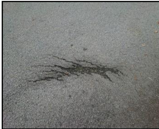
Figure 9: Rutting of pavement due to cyclic moisture changes, adapted from Daniel [21].
