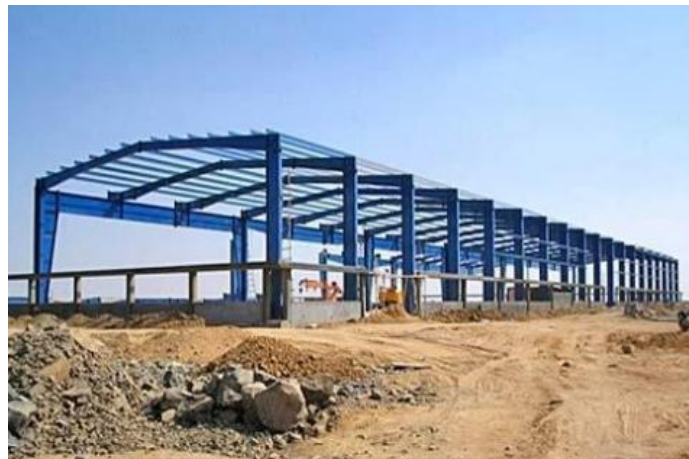
Fig. 2 On-site view of Pre-Engineered Building (PEB)
