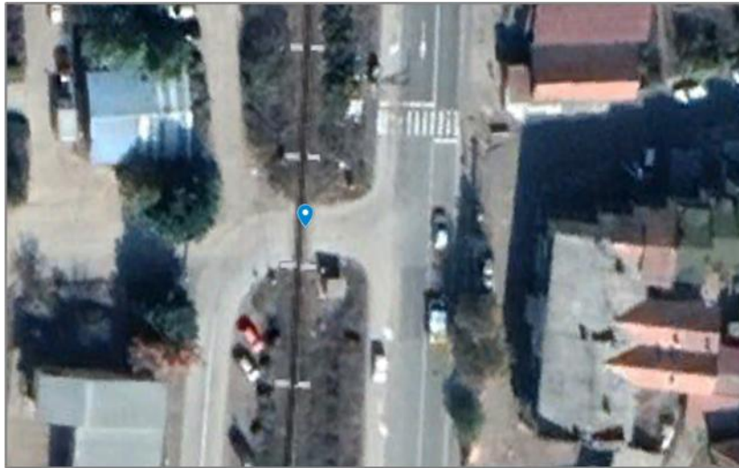
Figure 1: Indicative railway level crossing along the examined railway line.
