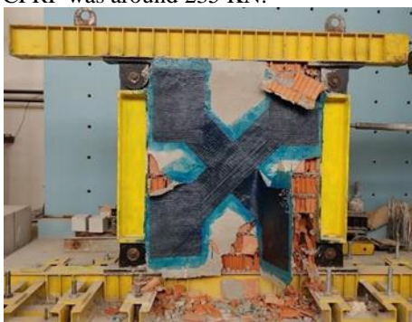
Figure 10. Damaged wall coated with CFRP
