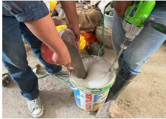
Figure 10. Mixing Foaming, Fine Aggregate, Cement, and Water
