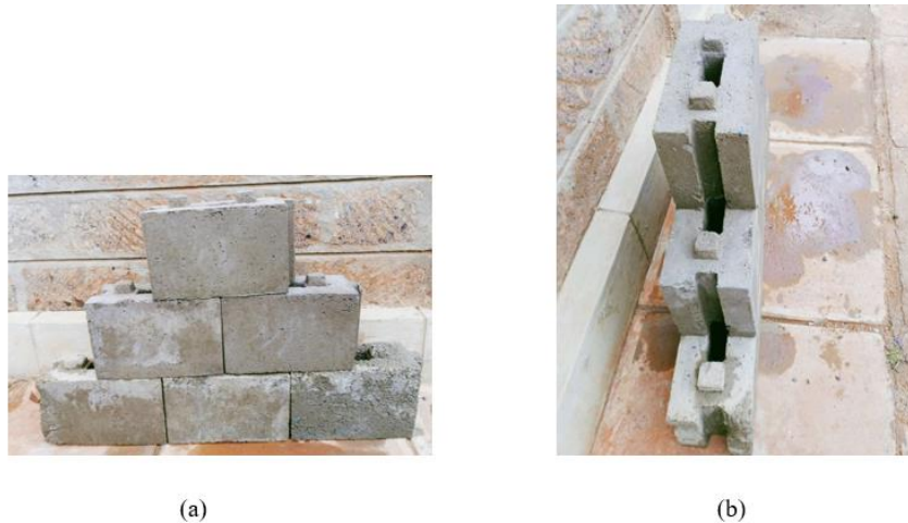
Figure 5: Front view (a) and side view (b) of a wall showing how the hollow blocks made using the fabricated mold interlock both vertically and horizontally.
