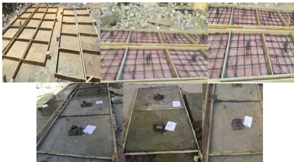
Fig4: Casting of FRGPC and OPCC slabs
