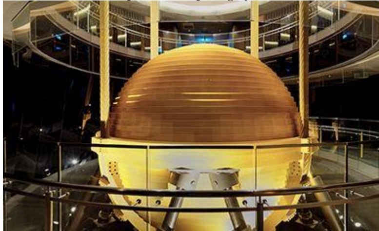
Figure 2 Taipei 101 Dampening System
