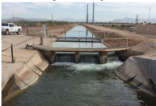
Figure 3. Vehicle and pedestrian bridges
