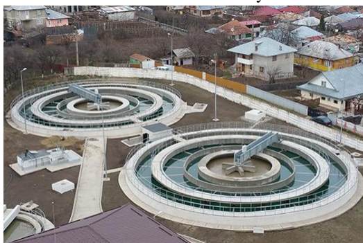
Figure 7. Example of water treatment works facilities in Vaslui city, Romania
