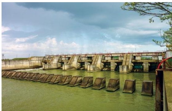
Figure 9. Downstream view of Zavoiiul Orbului Dam
