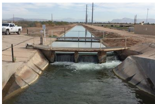
Figure 3. Vehicle and pedestrian bridges
