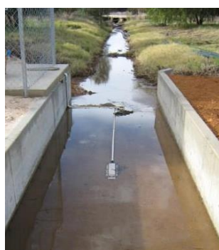
Figure 5. Canal discharge measurement telemetry system
