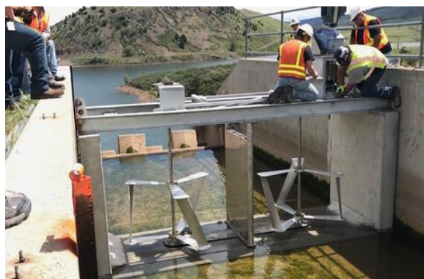
Figure 4. Placement hydrokinetic turbines in a irrigation canal
