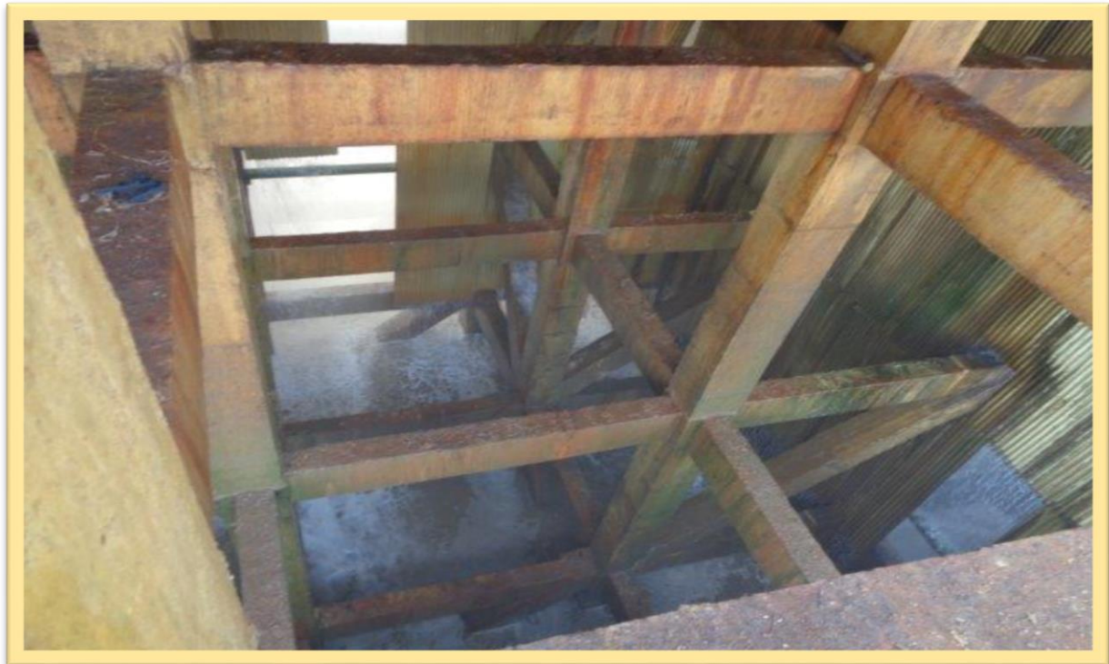
Picture 1 - CONCRETE CT WALLS WITH EPOXY COATING /FIBRE SHEETS/ WATER BASIN
