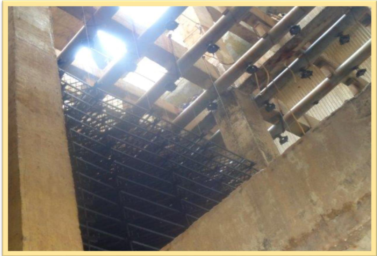
Picture 2 - CONCRETE CT WALLS WITH EPOXY COATING /FIBRE SHEETS/ WATER BASIN.
