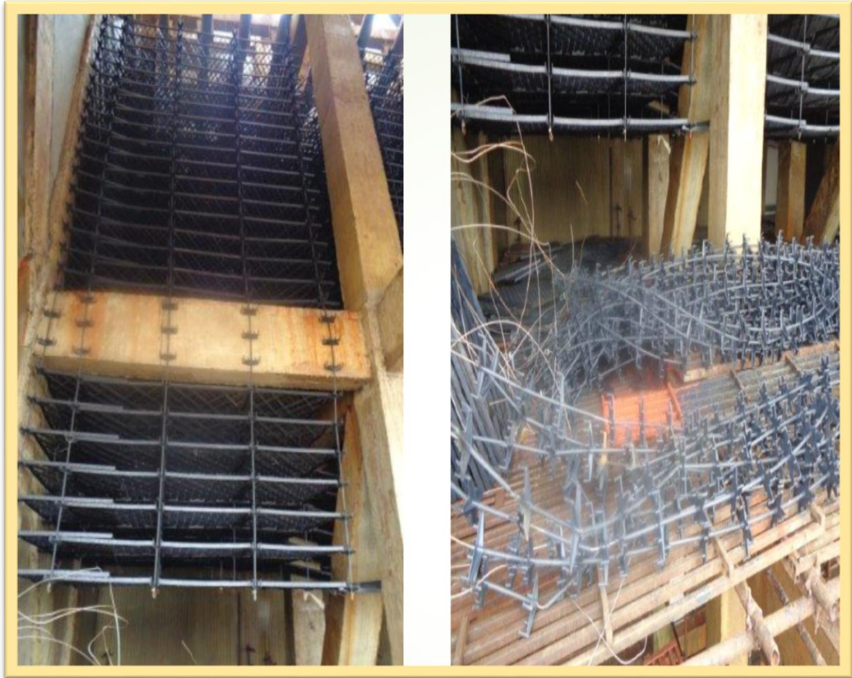
Picture 3 : FILLS STRUCTURE & SS WIRE/SPACER PIPES/SPIDERS
