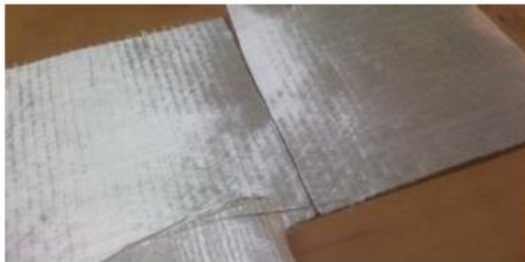
Fig.5: Demarcations and cutting of fiber cloth
