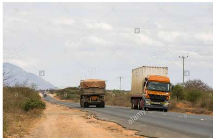
Fig. 2: Section of Voi - Maungu Road
