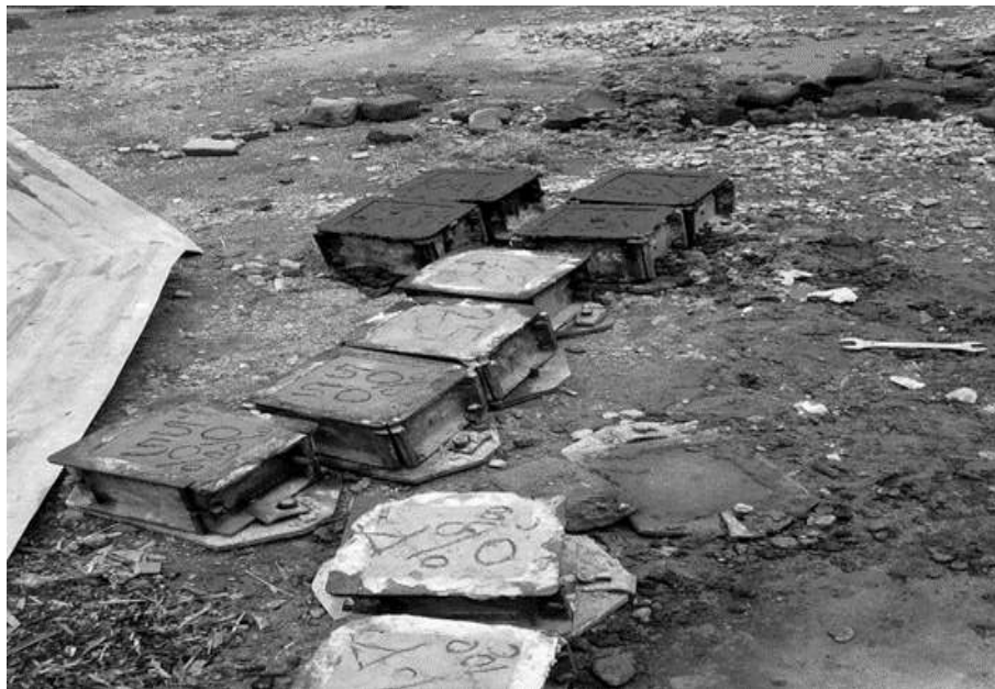
Figure 4: BLA/OPC Concrete Casting Section
