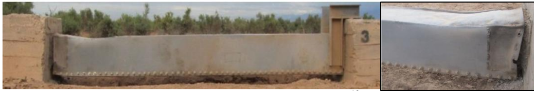
(c) Experimental failure shape 12
