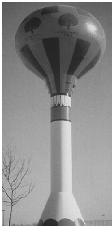
Fig3. Spherical cell storage tank
