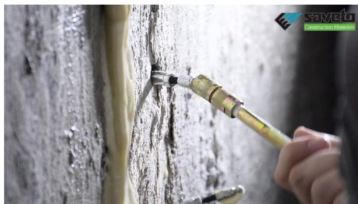
Figure 10. Show treatment of cracks by injection method
