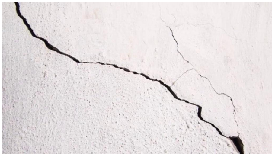
Figure 2: Typical elastic shrinkage cracks in an unreinforced concrete slab.
