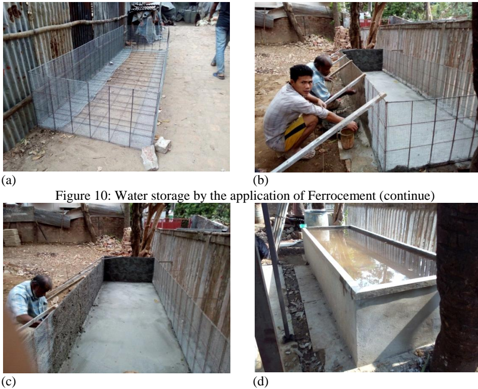
Figure 10: Water storage by the application of Ferrocement
