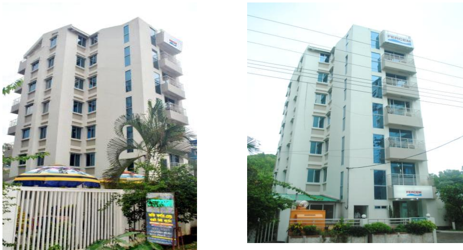
Figure 9: Cast-in-situ Ferrocement non-structural element work
