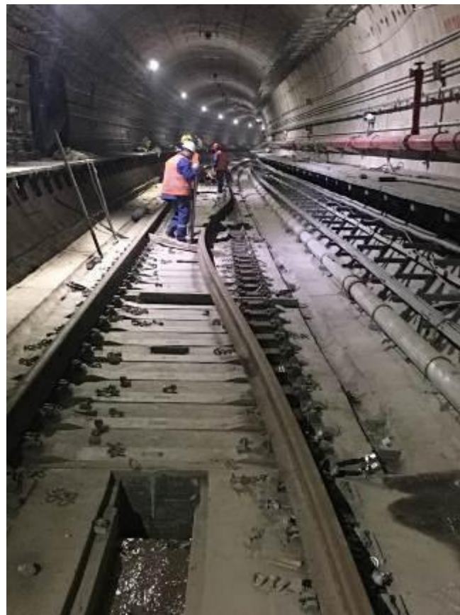
Fig 6 Bending the rail outward away from rail joint with 30m
