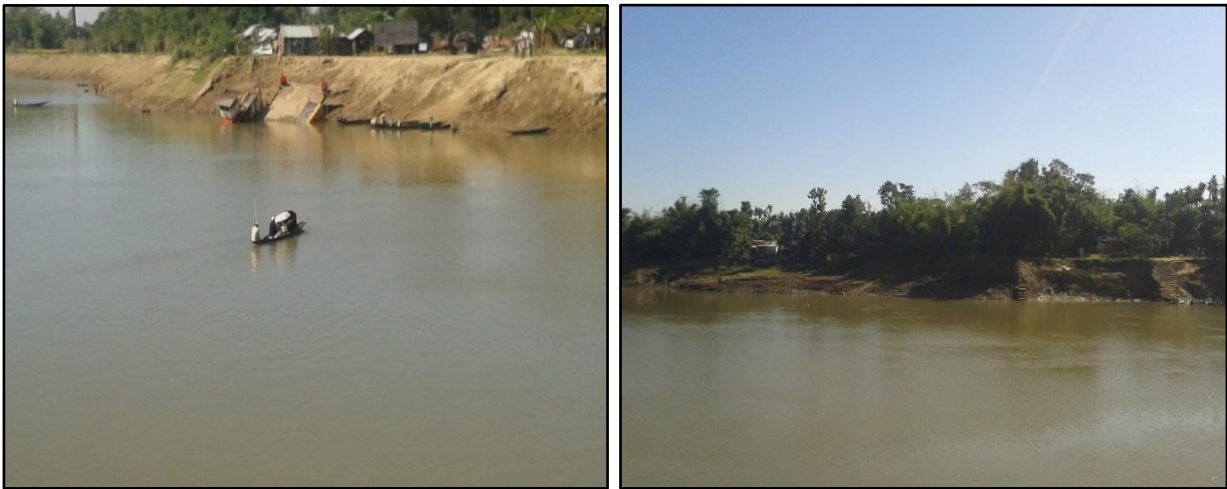
Figure: The proposed bridge location on the Kushiara river at Golapganj.
