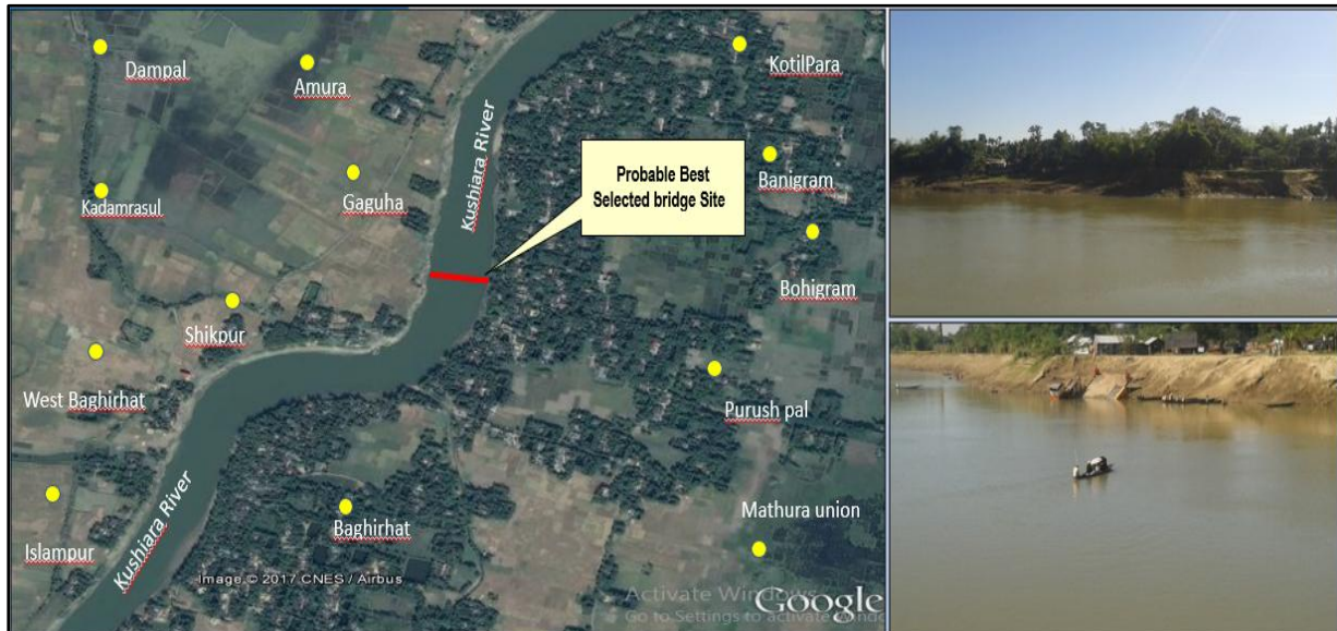
Figure: Proposed bridge location (Golapganj Bridge)
