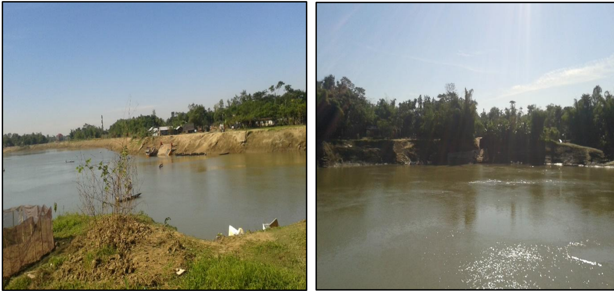
Figure: Left and right bank of the river at the bridge location with the harbor entrance for Kushiara river at Golapganj
