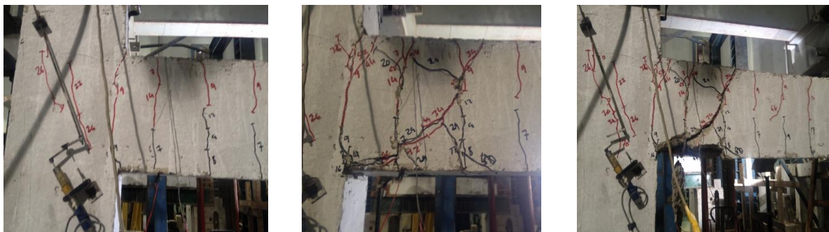
a) S1, shear failure attached with spalling of concrete due to yield of bottom reinforcement
