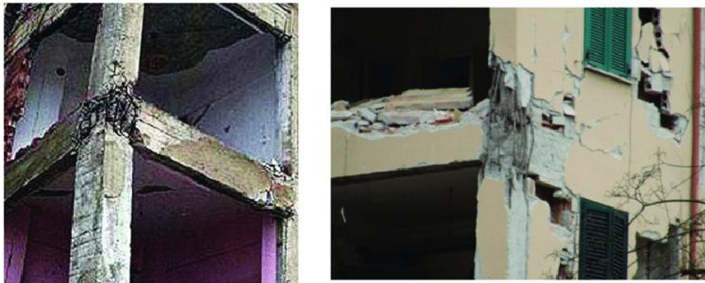
Fig. 1: Failure-of-corner-beam-column-joints-in-Izmit-earthquake-in-Turkey
