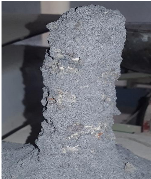
Figure 3: Bulging of ordinary Stone Column
