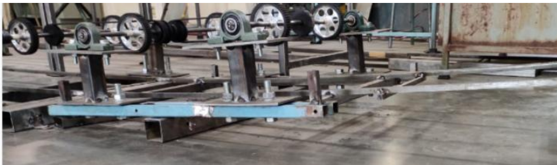
Fig. 6: Construction of ramp-up track
