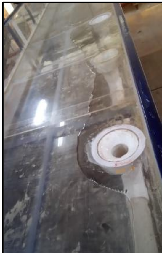
Fig.(17)Water receding in the transverse direction
