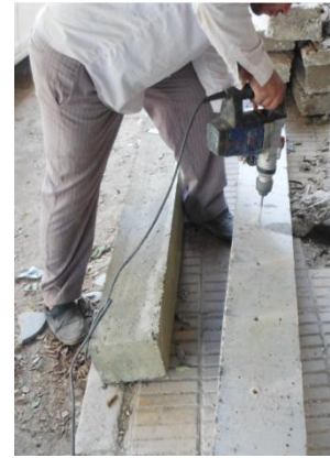
b) Positioning of the shear connector and drilling
