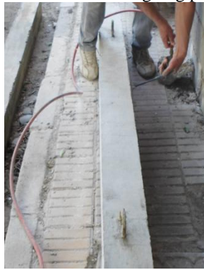
a) Surface Roughing process
