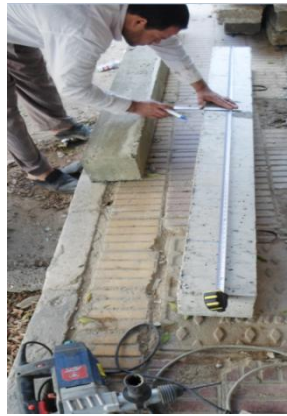
b) Positioning of the shear connector and drilling
