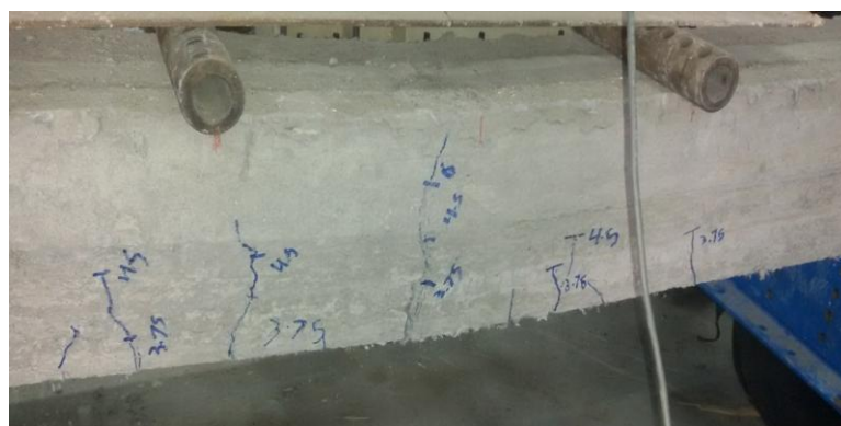
Figure 10 Strengthened beam (P-B) Cracks Pattern
