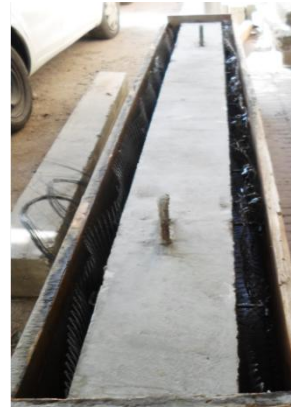
g) (FE-C- B) Beam ready for casting the 5 cm strengthening concrete
