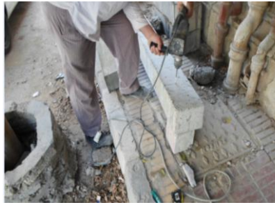
b) Drilling shear connector
