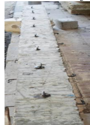
b) Positioning of the shear connector and drilling
