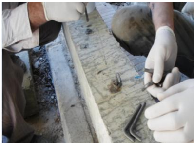
d) Mixing of the epoxy grout and implanting shear connector
