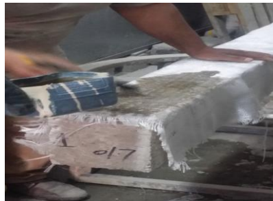
b) Glass fiber polymers sheets used in Strengthening
