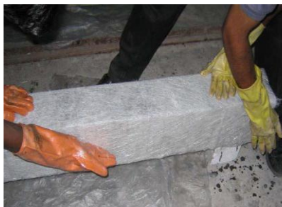
g) Strengthening with four layer of glass fiber polymers sheets
