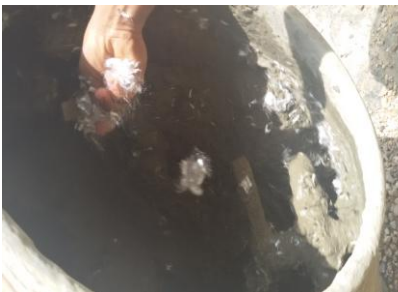
g) Mixing new concrete mix of polypropylene fiber
