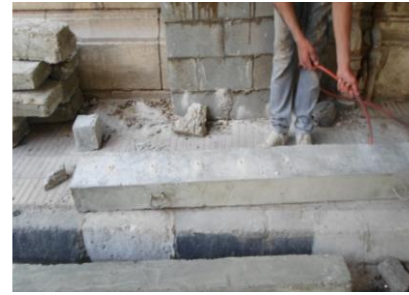
c) Using air compressor to remove dust and fines
