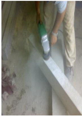
a) Surface Roughing process
