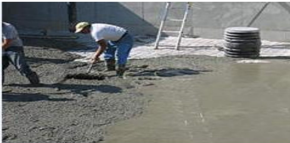
Fig. 1- Construction of horizontal joint [1]
