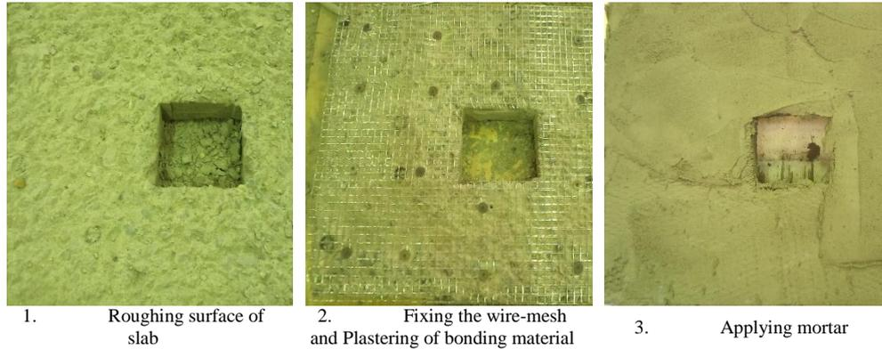
FIGURE 3. STRENGTHENING PROCEDURE
