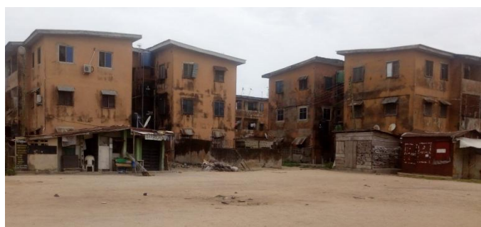
Plate 2: Illegal Installation of Air Conditioners, Television Decoder Signaling System, Water Tank
