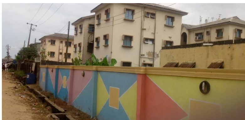
Plate 3: New Blocks of Flats in Iba Housing Estate
