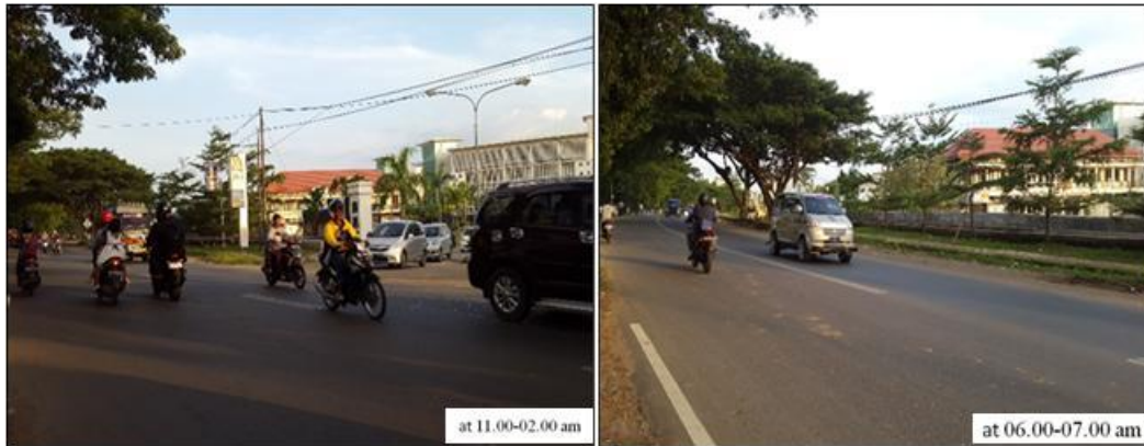
Figure 2. Existing condition of the Malino axis road in front of the Faculty of Engineering Hasanuddin University Gowa
