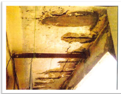
Figure 1.2 Corrosion of steel and Spalling of concrete in a RCC canopy.
