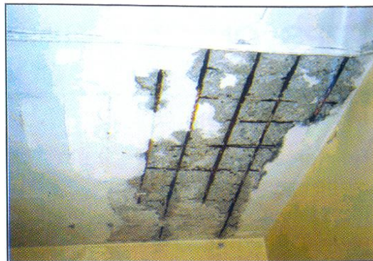
Figure 1.2 Corrosion of steel and Spalling of concrete in a RCC canopy.
