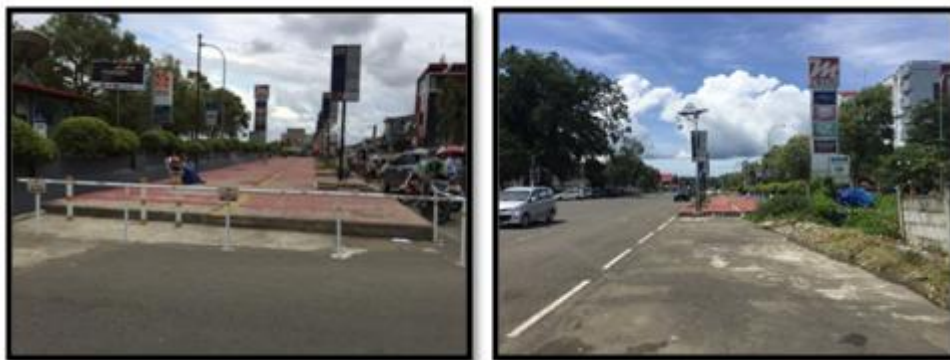
Figure 2. The pedestrian lane on the road Segment 1
