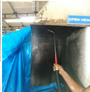
Fig. 15: Cleaning with chemicals
