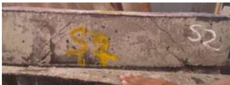
Figure 19 – Failure of reinforced concrete beam provided with externally bonded GFRP wrap
