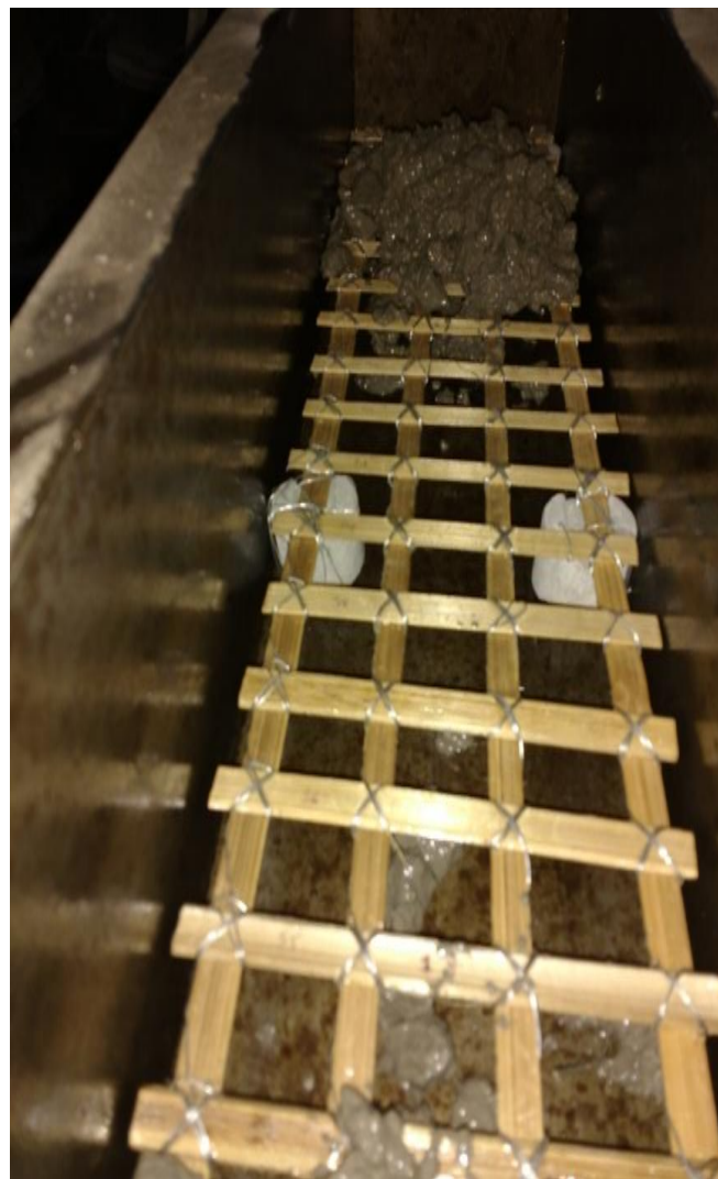
Figure 5: Bamboo-strip-mat Arrangement in Beam (1 mat)
