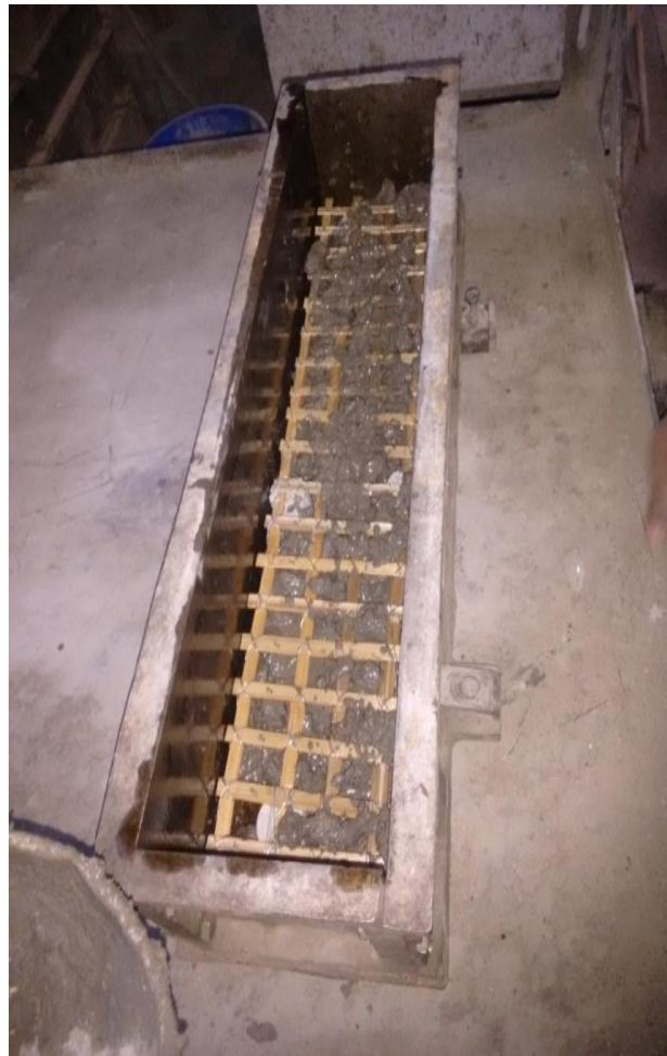
Figure 6: Bamboo-strip-mat Arrangement in Beam (2 mat)
