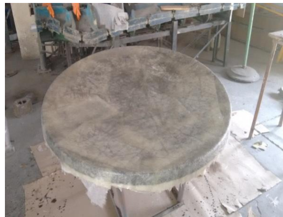
Fig 5.2: laying of fiberglass reinforcement
