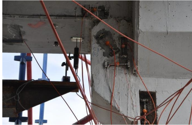
Fig. 9 photo of fixation displacement and inclinometers for interior and external beams.
