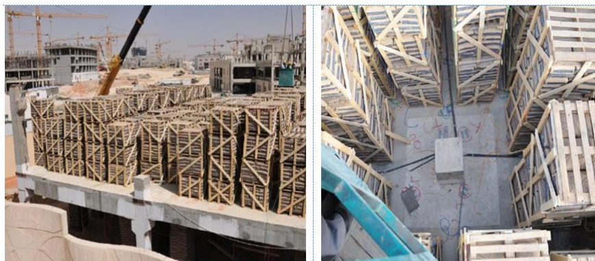
Fig. 6 Loading of the Mockup Structure
