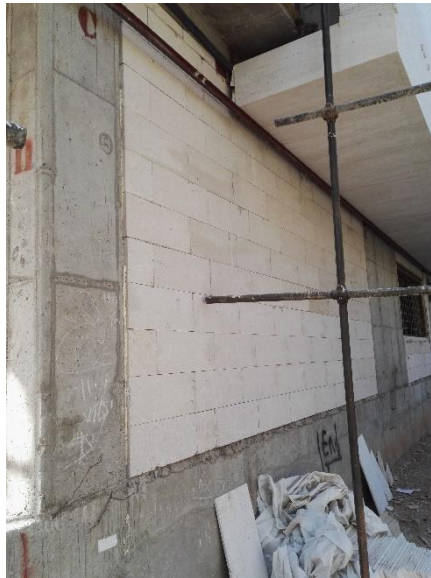
Fig1. Wall with AAC material in a reinforced concrete frame
