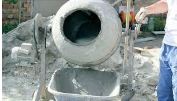
Fig2 it shows the concrete machine mixer.
