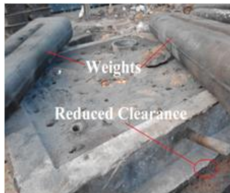
Fig.17. Heavy Weights on Cope
