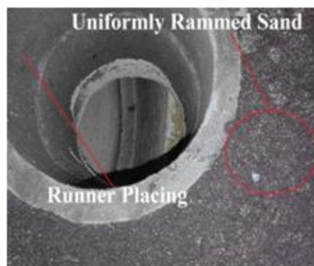
Fig.13. Sand Ramming and Runner Placing
