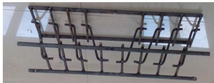
Fig.1. Reinforcement of Beam SSB
