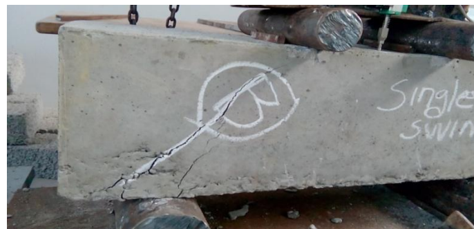
Fig.7. Crack Pattern of SSB
