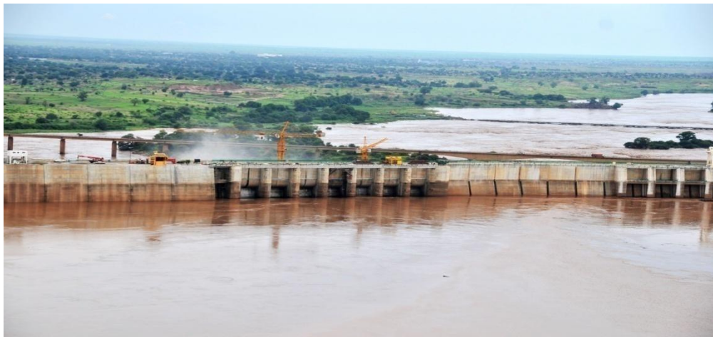
Figure (1) Roseires Dam Concrete Section upstream view
