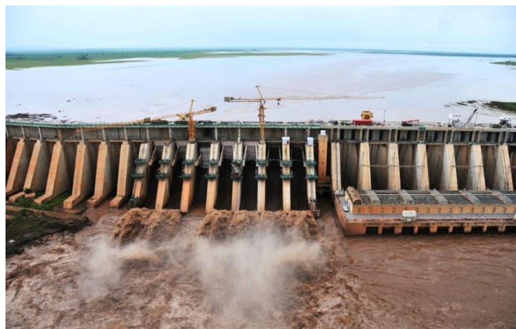
Figure (1) Roseires Dam Concrete Section downstream view
