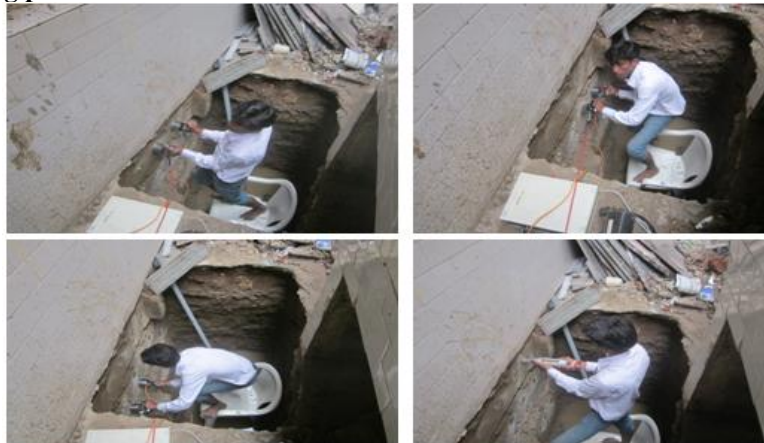
Fig 5. Performance of UPV & Schmidt rebound hammer test
