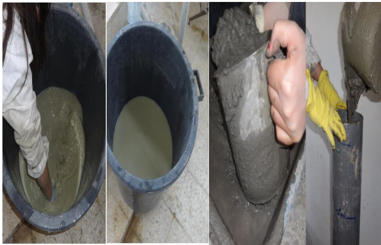
Photo 2. Bentonite dosing Preparation
