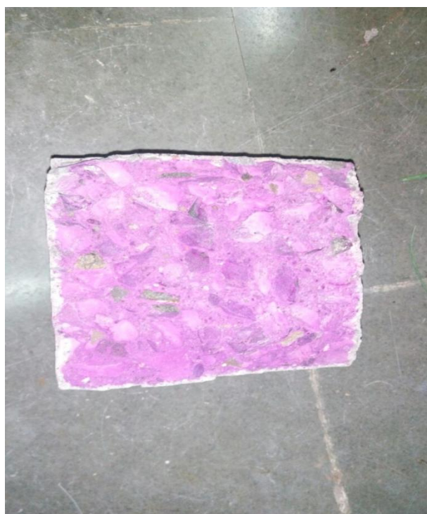
Fig 3 : Carbonation test using phenolphthalein indicator.
