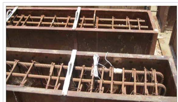
Fig.4.2.1 (b) Steel Formwork
