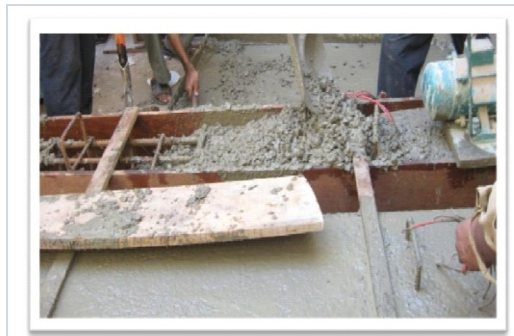
Fig.4.6.1 Casting of Beam Specimen
