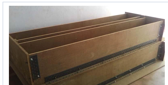
Fig.4.2.1 (a) Wooden Formwork
